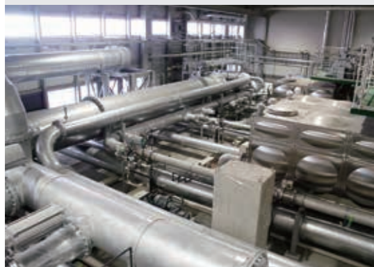
Maximum 50D upstream straight pipe for accurate calibration
