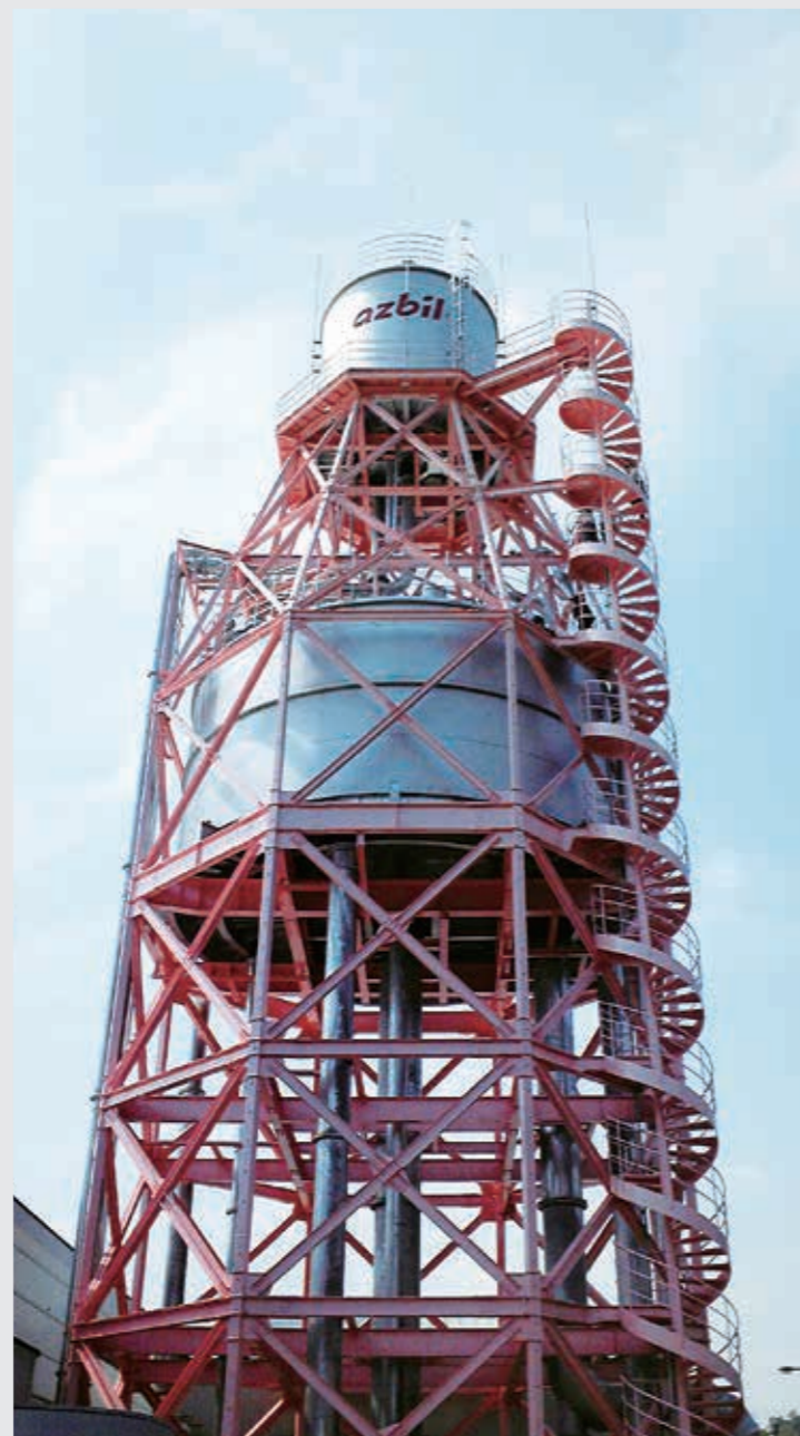
Elevated water tank for calibration
